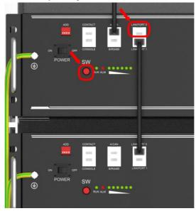
5) Press the **red SW button** of **master battery** to power on, all the battery LED light will be on one by one from the Master battery:
